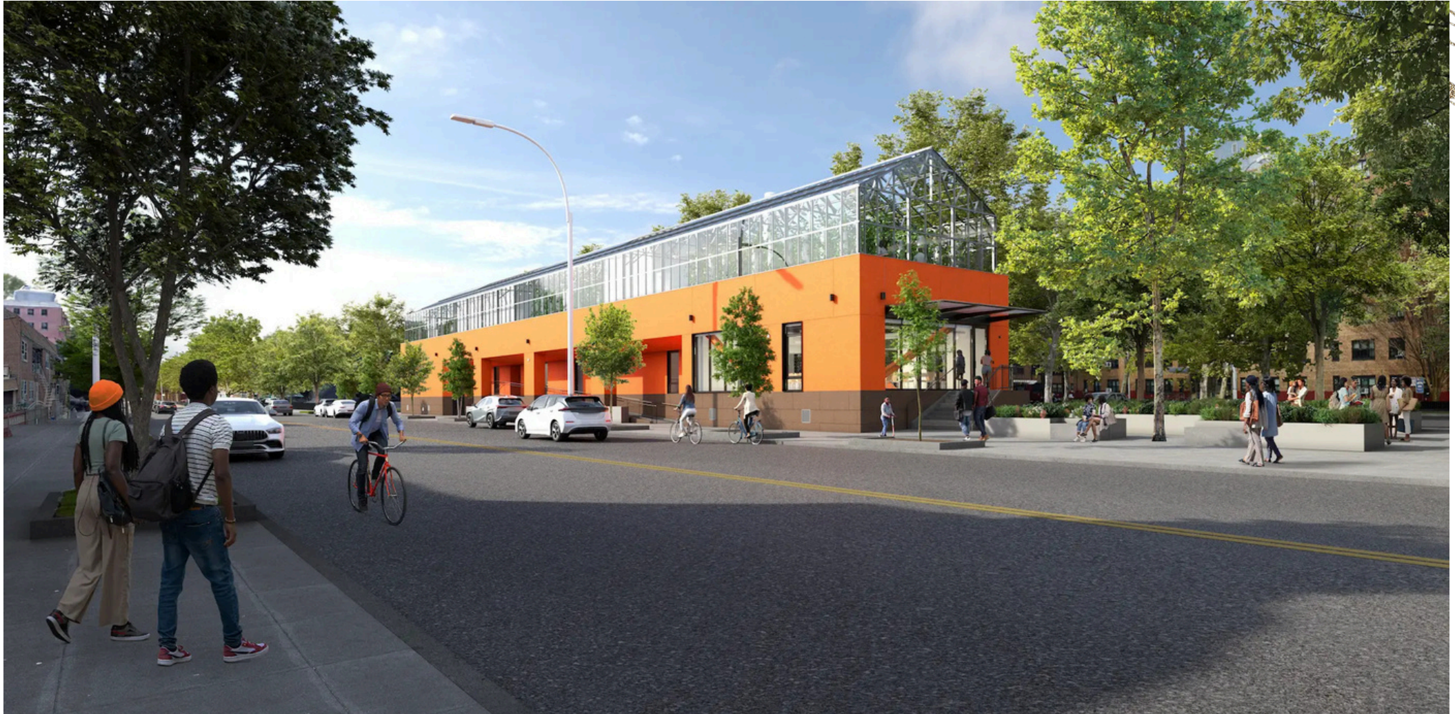
9,900 SQFT BUILDING - MARLBORO AGRICULTURAL EDUCATION CENTER (MAEC), VIEW FROM WEST 11TH STREET. (COURTESY STUDIO GANG)
